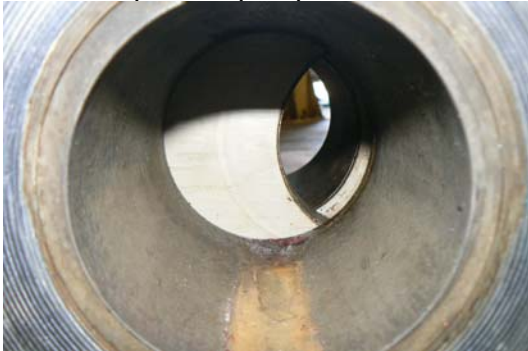
Scale removed without damage to sealing surface
